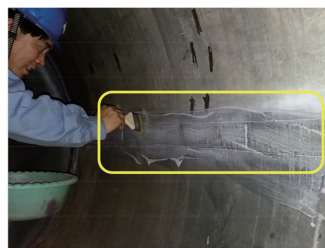
(c) 覆层盖板侧刷肥皂水检漏
