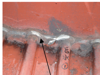
(c) 焊缝中间穿孔处理：打磨
